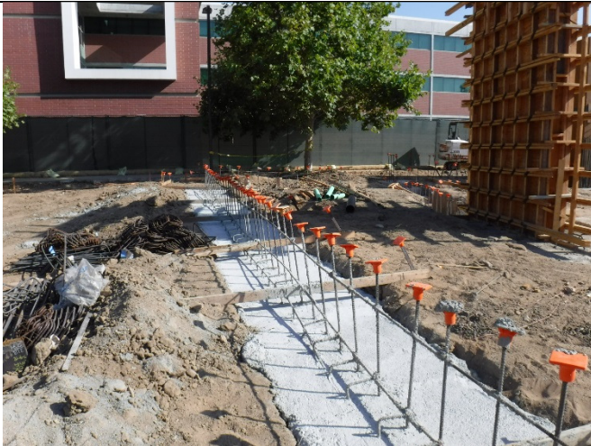
Photograph 3. Vertical rebar and steel form stakes were properly capped to protect against impalement. This is an ongoing item.
