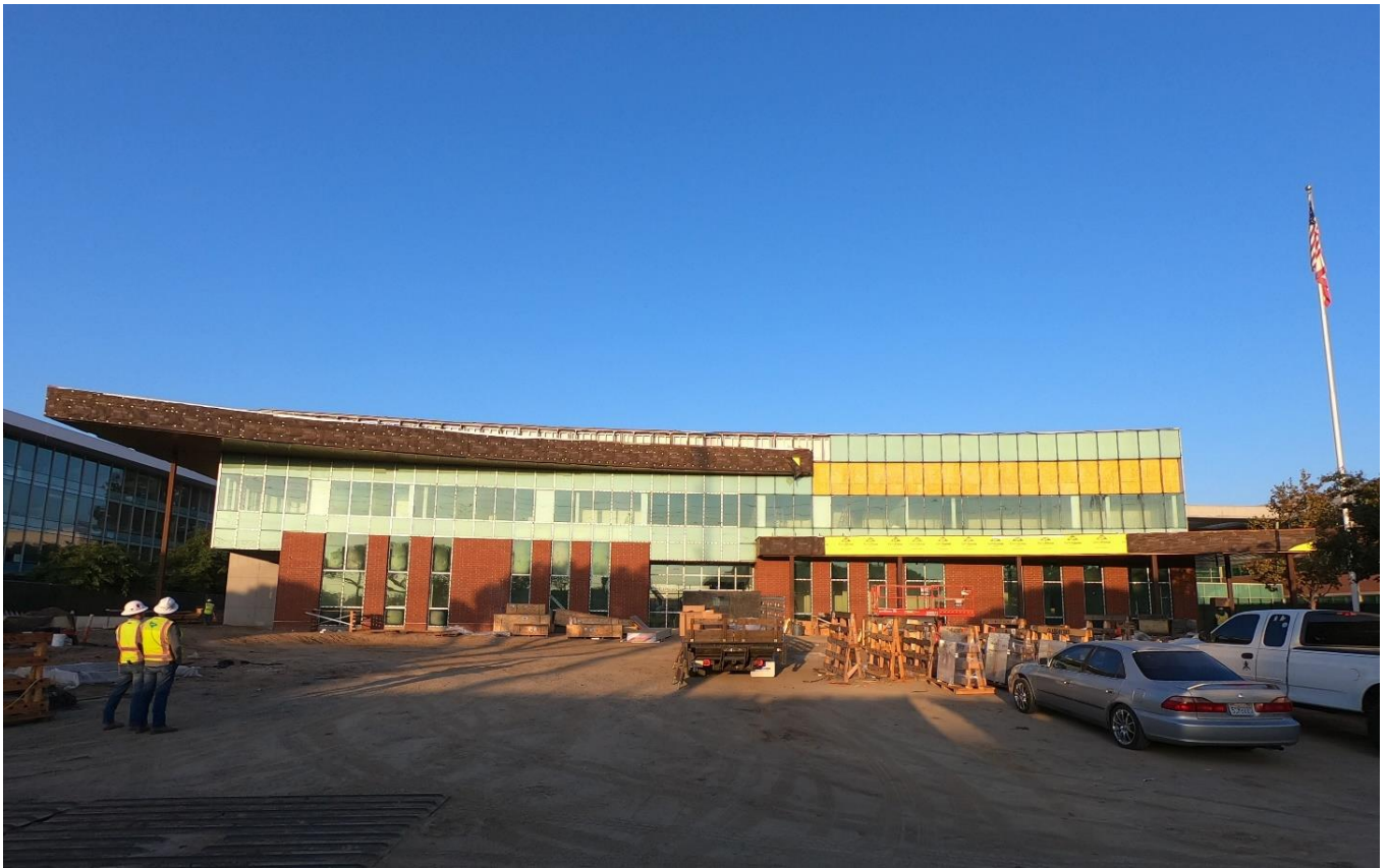
Admin – East Main Entrance
