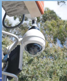
2008: Security Cameras Installed
