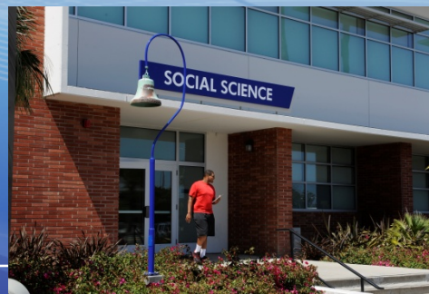
2011: Social Science Building Renovation
