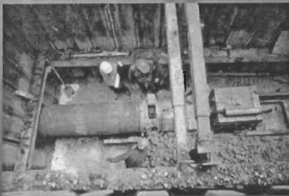
Open Pit over a Sewer
