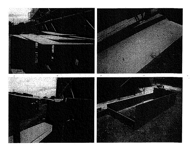
2. Steel Window Surround/Fin installation started on north end of the EAST elevation. It was observed that the shade fin is on the NORTH side of the window. The shade fin shall be installed so that fin is on the SOUTH side of the window, providing shade to the glazing. The shade fin shall be constructed and installed per the approved contract documents and details as the opposite hand. See partial plans and elevations below.
