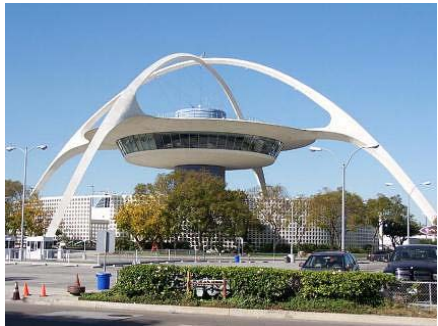
Iconic central restaurant/tower
