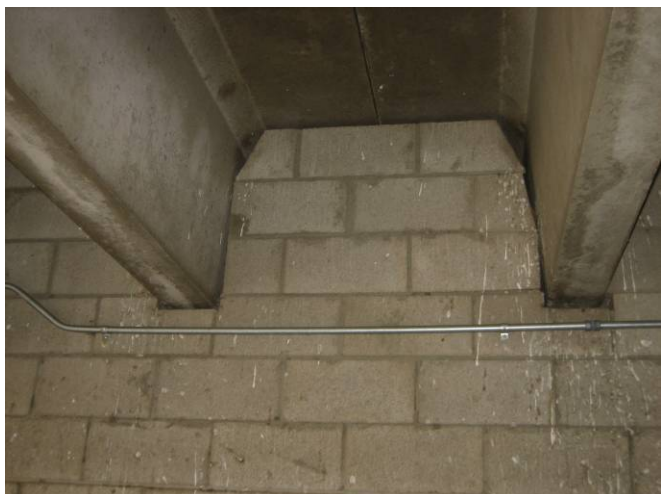
Photo C32: Inadequate Gap at Double Tee/Wall
