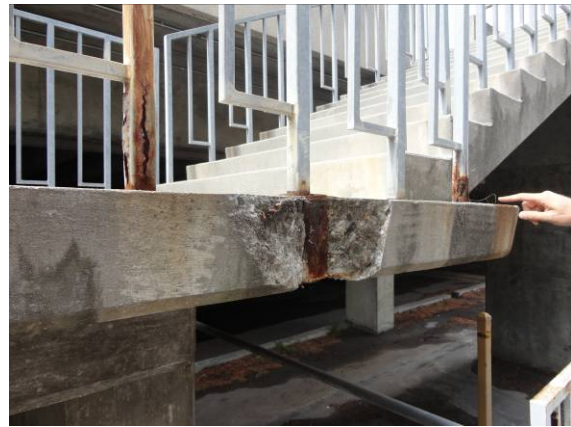
Photo # 44 Railing rut and concrete spalling
