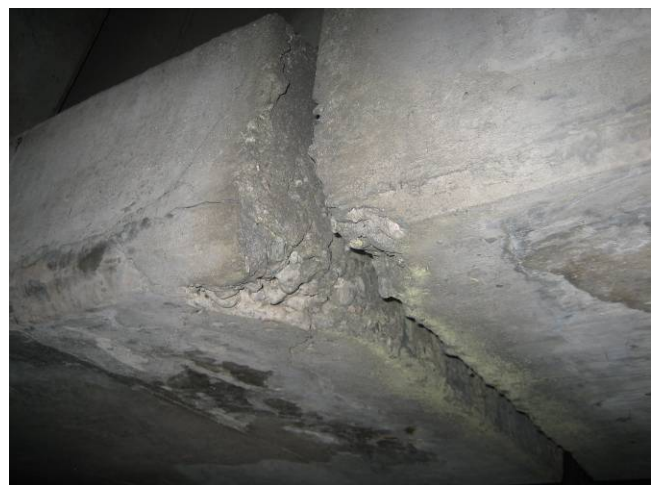
Photo C24: Poor Concrete at Girder
