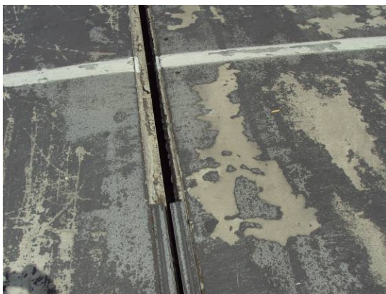
Photo # 28 Deteriorated expansion joint.
