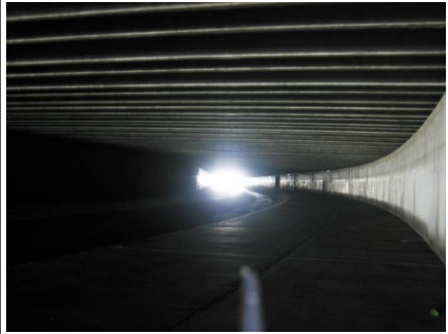
Photo C62: Typical Double Tee over Channel
