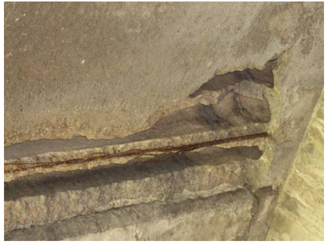
Photo C8: Slab Spalling/Deteriorated Reinforcing
