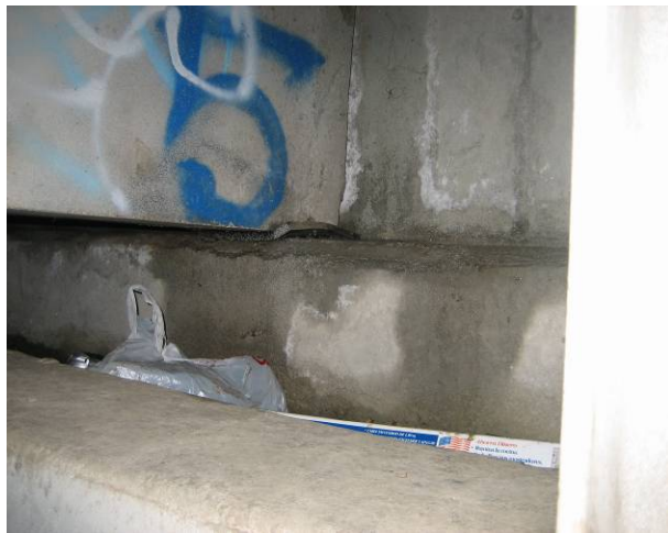
Photo C63: Double Tee Support over Channel
