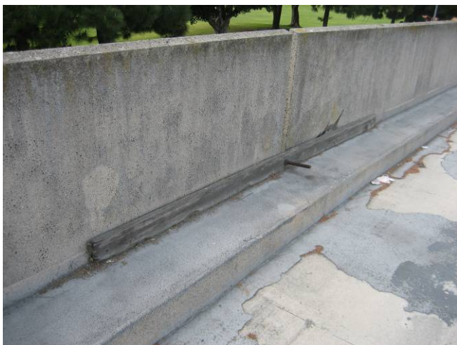
Photo C53: Damaged Wall Support
