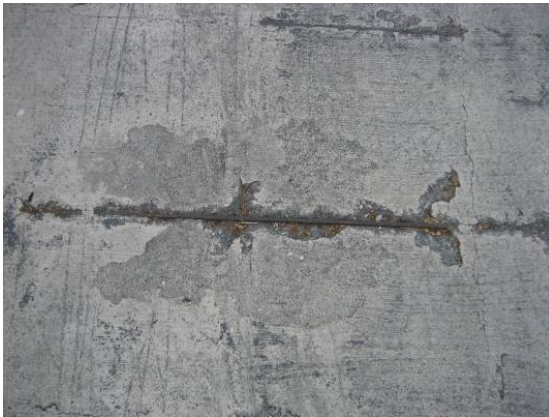
Photo # 20. In numerous places, rebars in the concrete topping at both levels are exposed and corroded leading to concrete spall as well
