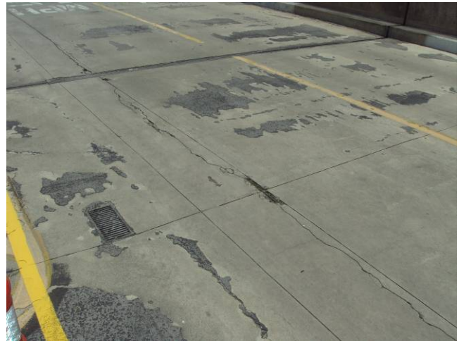
Photo C44: Typical Slab Cracking at Girder
