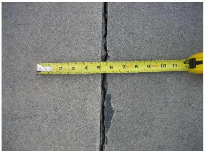
Photo C42: Typical Control Joint
