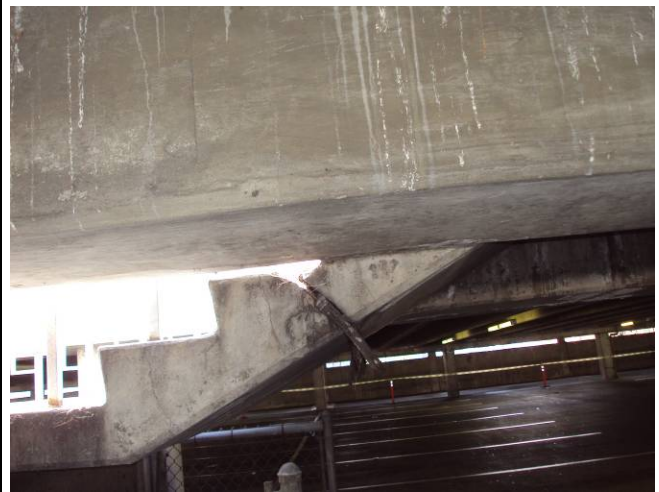
Photo B24: Stair Concrete Stringer Damage
