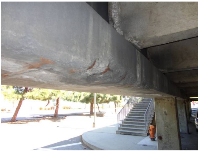
Photo C19: Girder Damage
