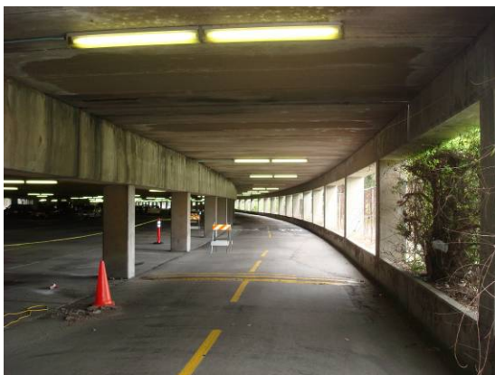
Photo # 14. Spalled concrete on the drive lane. The entire bottom surface of the upper deck is stained and wet.
