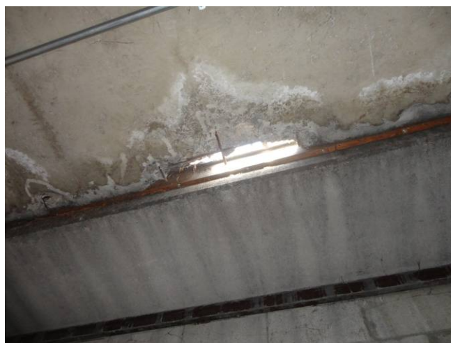
Photo C35: Slab Deterioration at South Ramp
