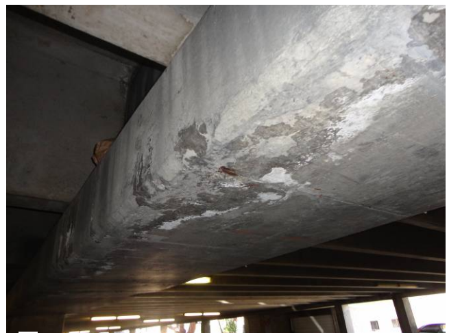
Photo C22: Girder Damage
