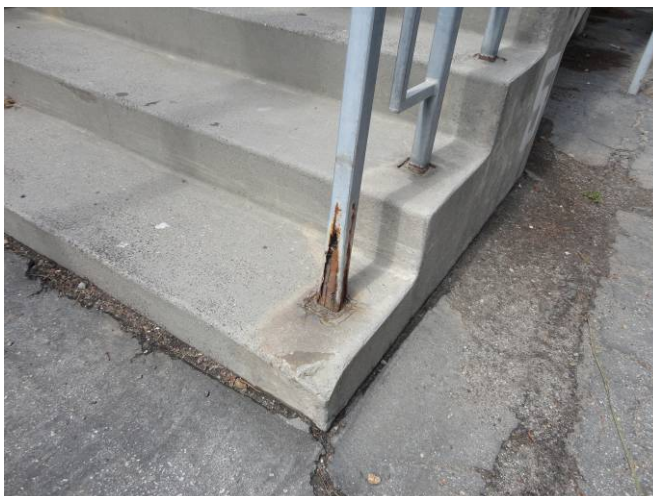
Photo A8: Stair Handrails Not Accessible
