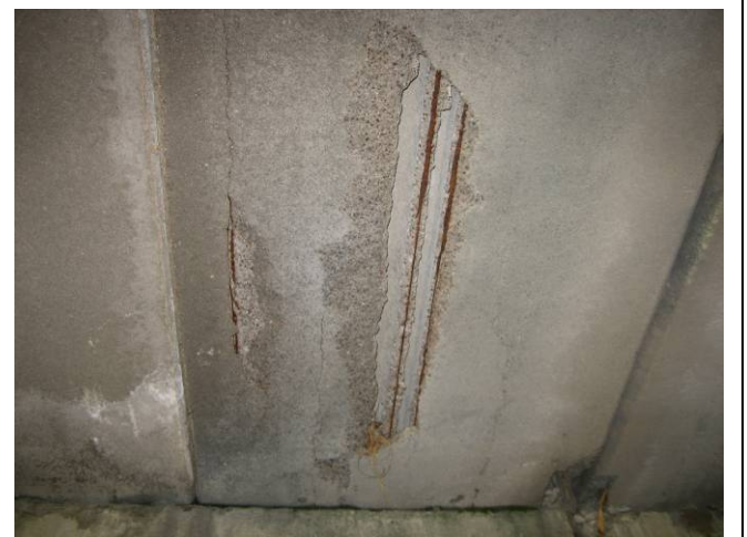
Photo C6: Spancrete Slab Damage
