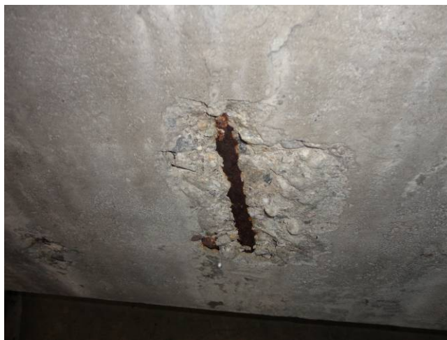
Photo C21: Girder Damage
