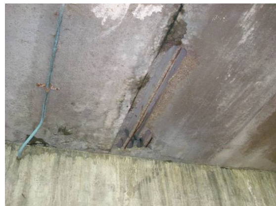
Photo # 15. Hollow cores are exposed. Concrete strength is compromised.
