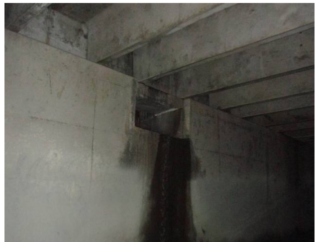
Photo C66: Double Tee Support over Channel
