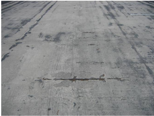
Photo C43: Exposed Slab Reinforcing
