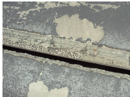
Photo # 42 opened expansion joints
