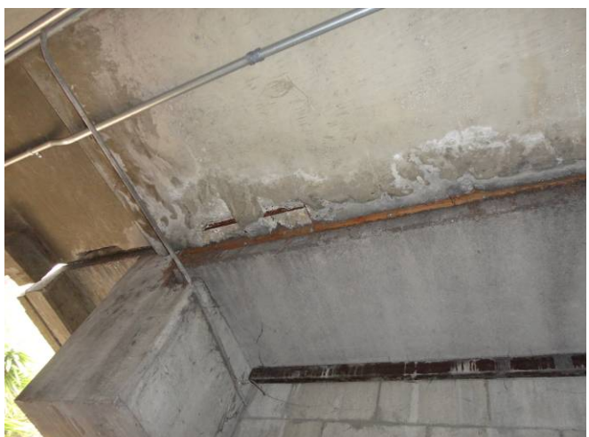
Photo C36: Slab Deterioration at South Ramp
