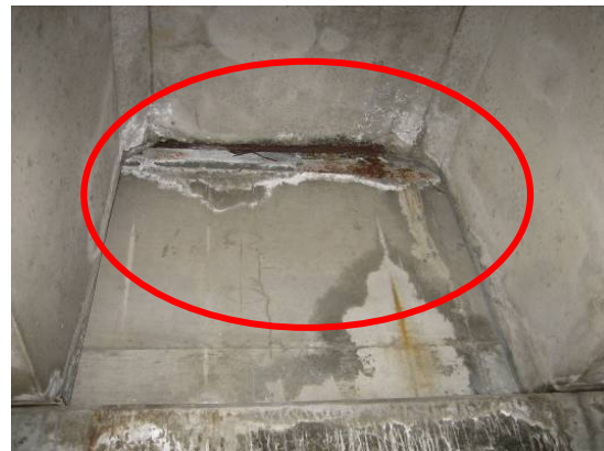
Photo # 19 Corrosion of rebars at the Double Tees Flanges.
