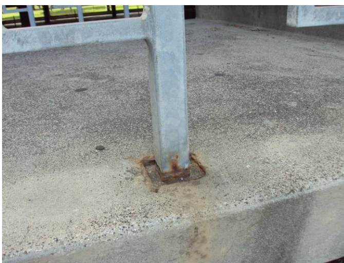
Photo A16: Stair Guardrail Rusting
