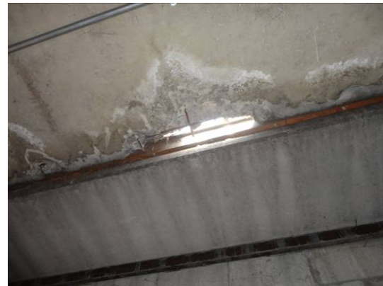
Photo # 31 Spalled concrete at the ramp joint
