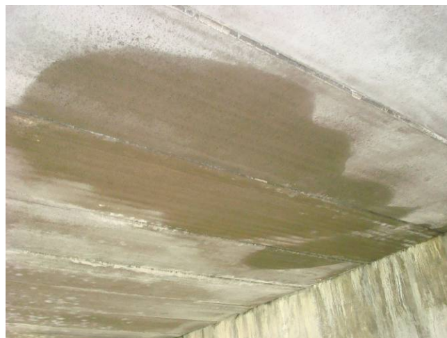
Photo C14: Typical Water Infiltration
