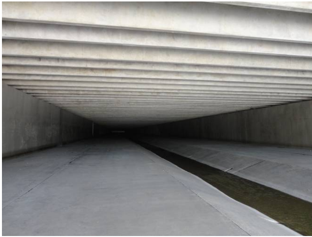
Photo C61: Typical Double Tee over Channel
