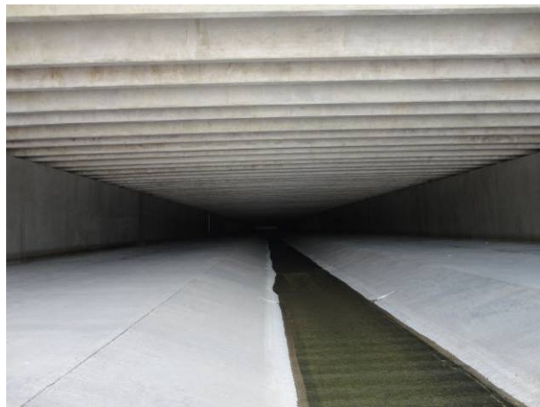
Photo # 4 Double-tee beams span across the Channel and provide parking at first level.
