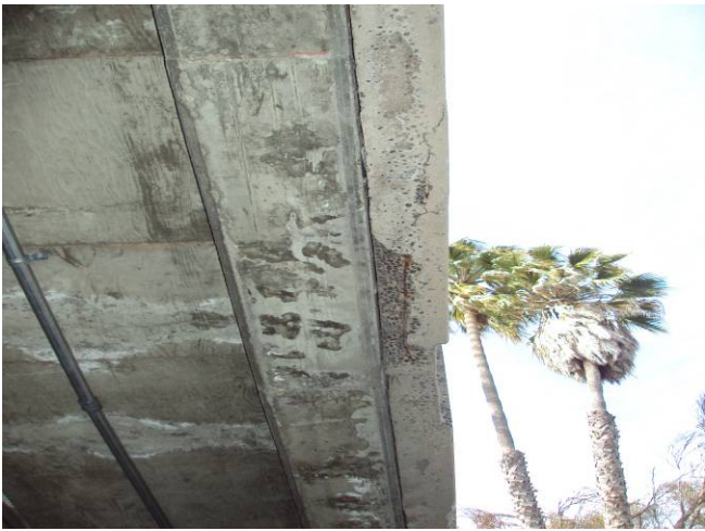
Photo B15: Precast Fascia Spall and Crack
