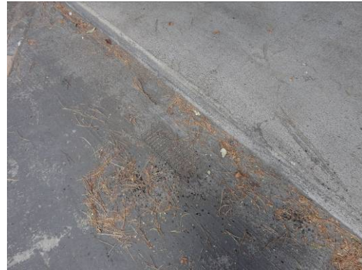
Photo # 28 Example of clogged drain- Grid Line D
