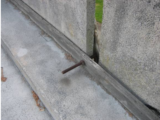
Photo # 34 Temporary Repair of Precast Joints
