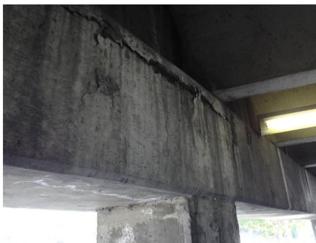
Photo C16: Girder Damage
