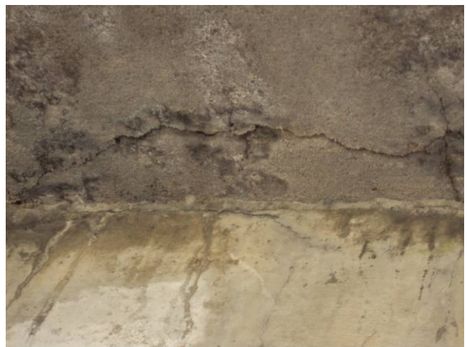
Photo C12: Typical Spancrete Slab Cracking
