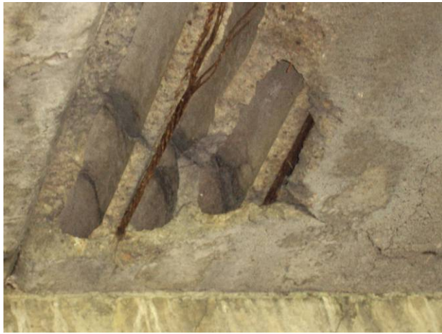
Photo C7: Slab Spalling/Deteriorated Reinforcing
