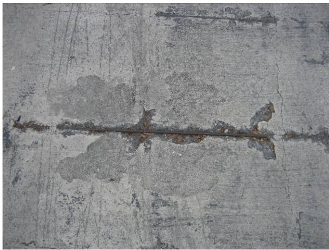
Photo C41: Exposed Slab Reinforcing
