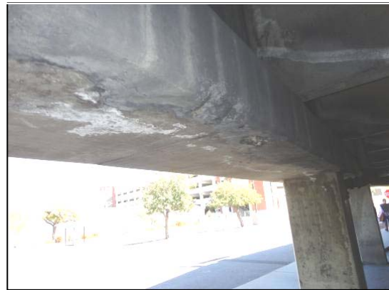
Photo # 23 Concrete spalling caused by water intrusion and rust of bottom rebars
