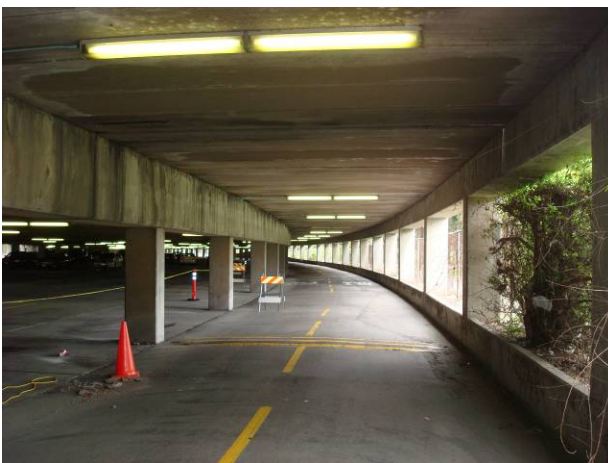
Photo # 6 The Western Drive includes two lanes for traffic circulation. Its 20ft span is covered by spancrete hollow core precast planks.
