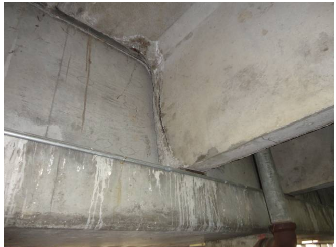
Photo C26: Typical Double Tee Seat Damage
