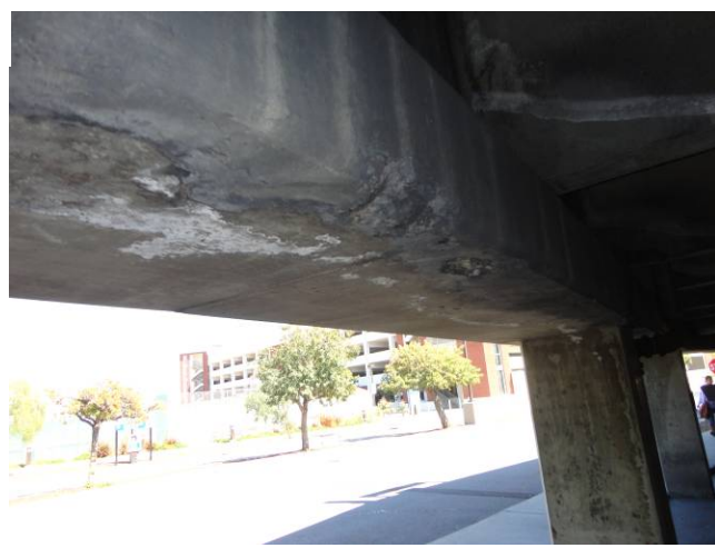
Photo C18: Girder Damage
