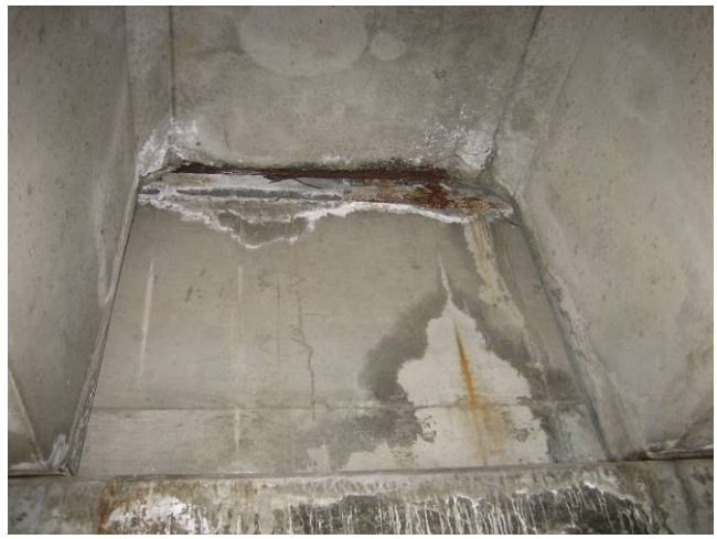
Photo C28: Typical Corrosion at Double Tee
