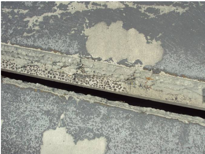
Photo B11: Damaged Expansion Joint
