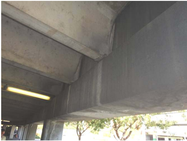
Photo C25: Typical Double Tee Seat Damage
