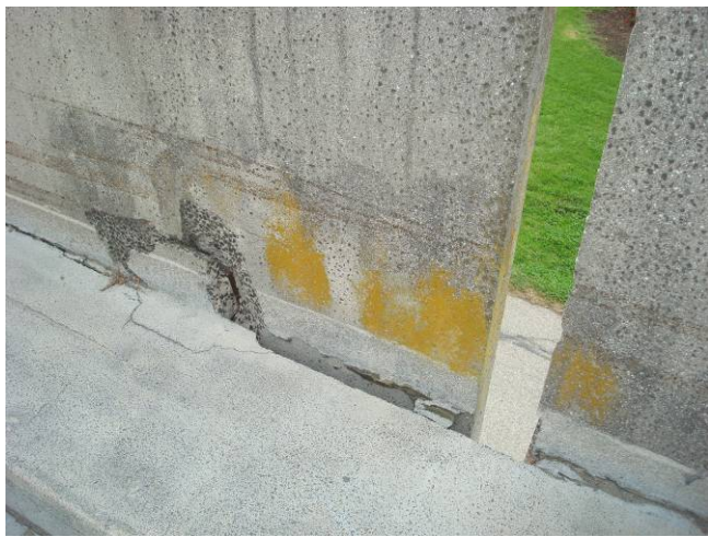
Photo C51: Damaged Wall Support
