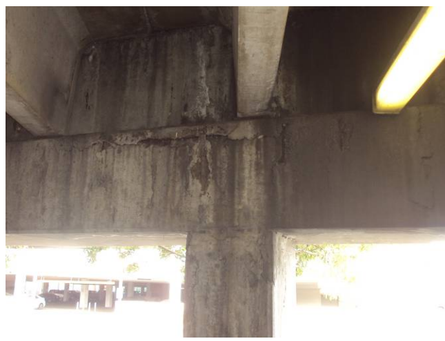
Photo C15: Girder Damage
