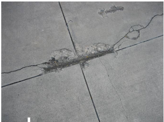
Photo C40: Slab Crack/Exposed Reinforcing
