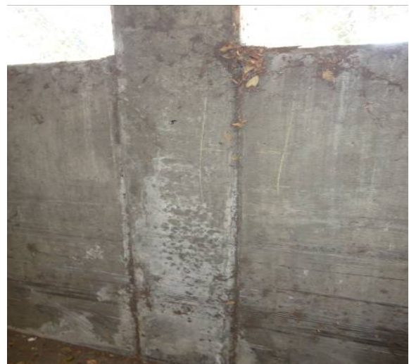
Photo C48: Cracks at Short Columns
