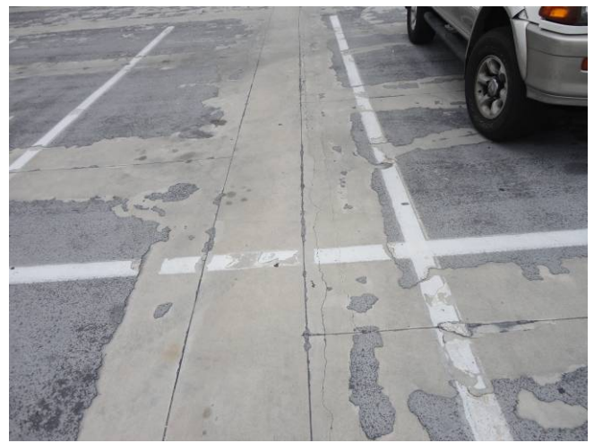
Photo C38: Typical Slab Cracking at Girder
