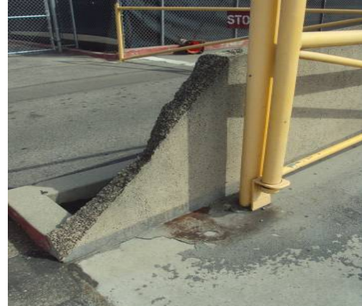
Photo # 35 Damaged Precast units
