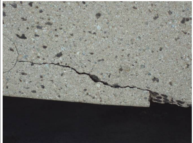
Photo B16: Precast Fascia Spall
