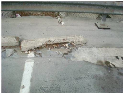
Photo # 41 Damaged Car Stops
