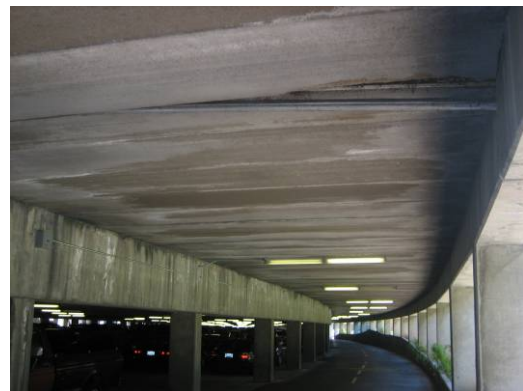
Photo # 27 Deteriorated joint at west drive
