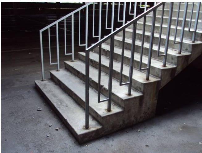
Photo B23: Stair Tread Concrete Spalling
