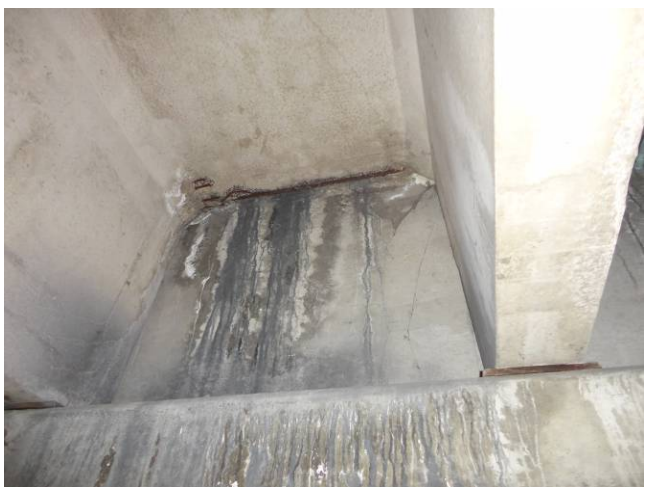
Photo C29: Typical Corrosion at Double Tee
