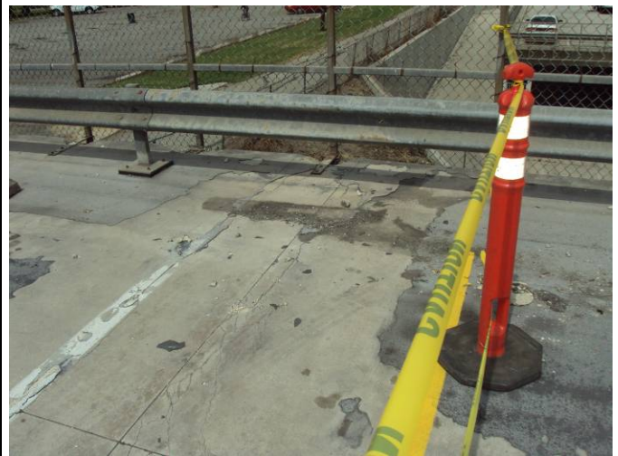
Photo B6: Waterproof Deck Coating gone
