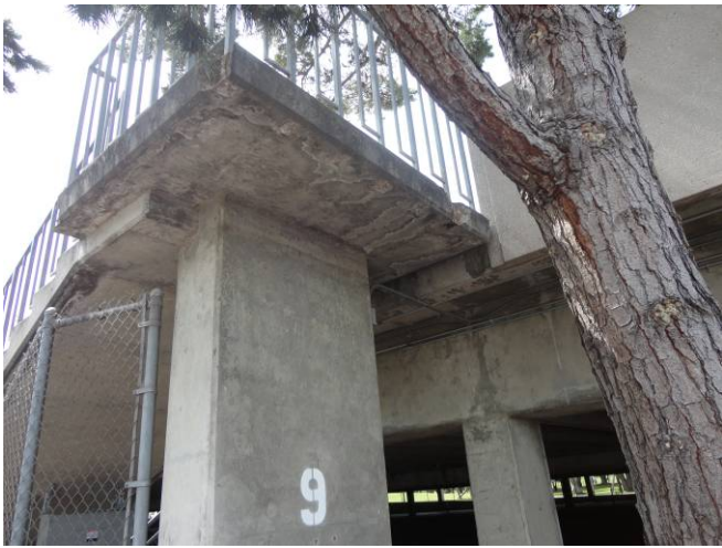
Photo B21: Stair Landing Concrete Spall
