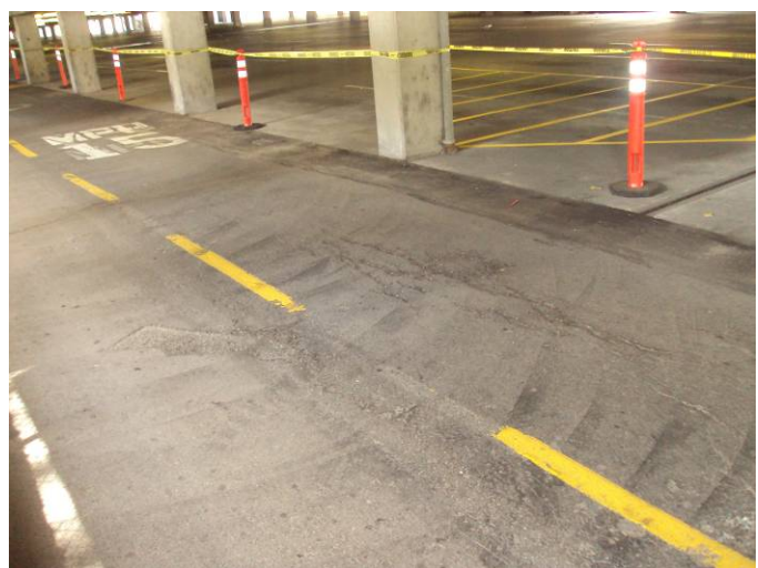
Photo A15: Asphalt Parking Tripping Hazard
