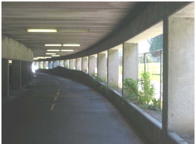
Photo C45: Short Columns at Drive Lane A-B
