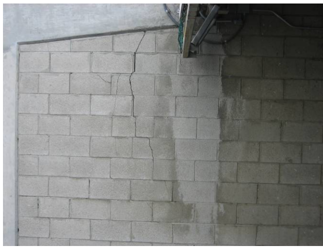
Photo C31: Crack at North Ramp Wall
