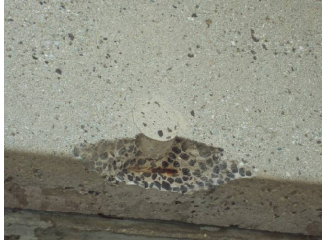
Photo B14: Precast Fascia Spall
