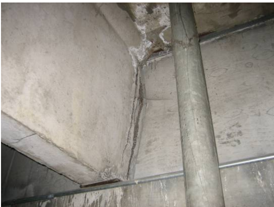
Photo # 18 Concrete cracking at the beam's end and signs of water intrusion.
