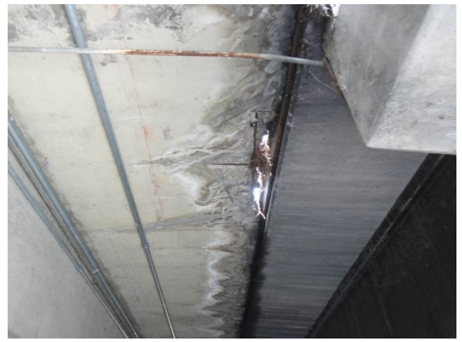
Photo C34: Slab Deterioration at South Ramp
