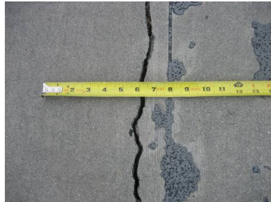
Photo # 21. Cracks up to one-quarter-inch wide are scattered on the top surface of the upper deck.
