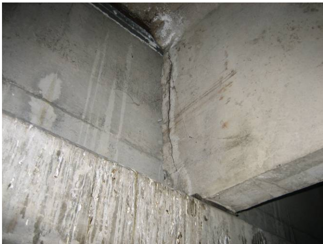
Photo C27: Typical Double Tee Seat Damage
