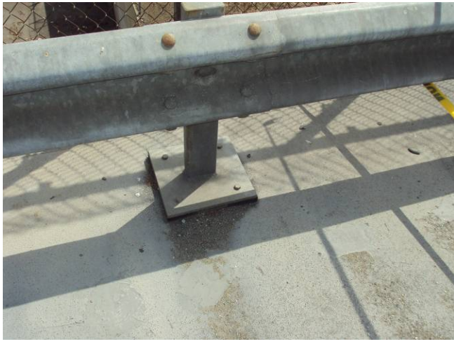
Photo B28: Chain Link Guardrail
