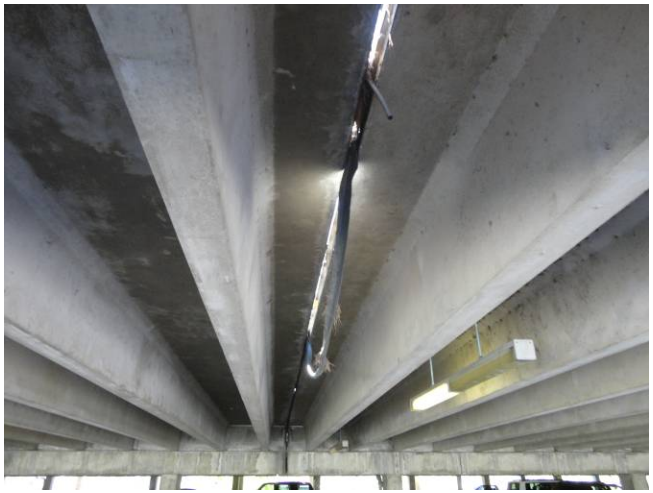
Photo B12: Damaged Expansion Joint
