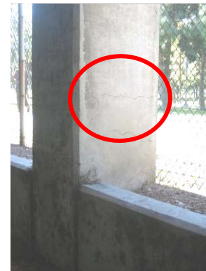
Photo # 33 Flexural cracks at short columns
