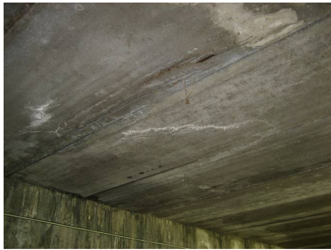
Photo C9: Typical Spancrete Slab Spalling
