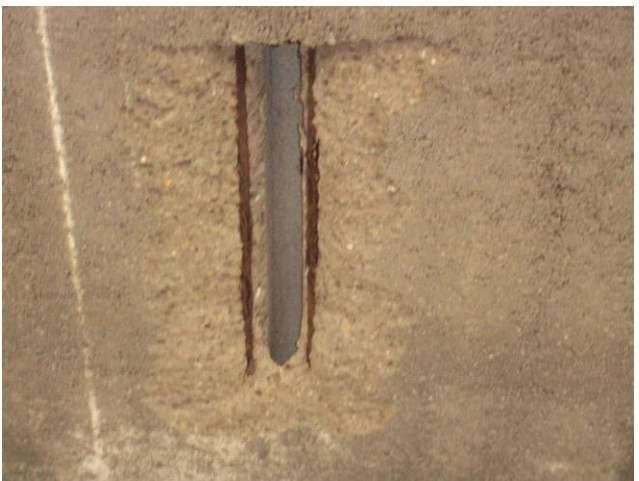
Photo B35: Hollow Core Slab Distress
