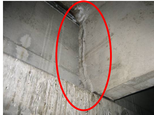
Photo # 17 Transverse cracks at the beam end.
