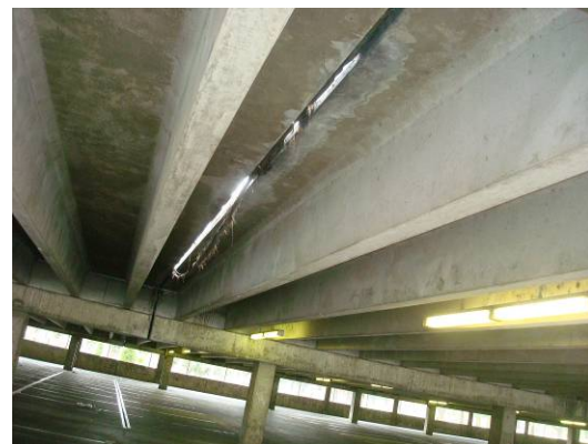
Photo # 29 Failed joints between the double-tee beams
