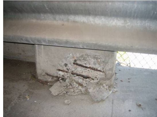
Photo # 25 Damage at the bottom of the column
