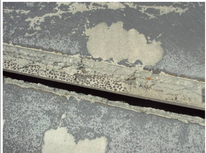
Photo A6: Expansion Joint Tripping Hazard
