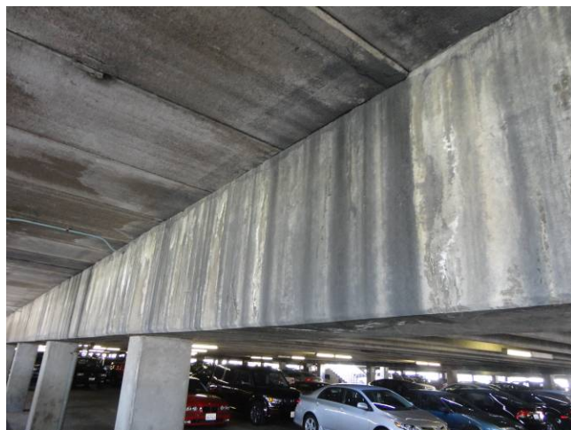
Photo C13: Typical Water Infiltration
