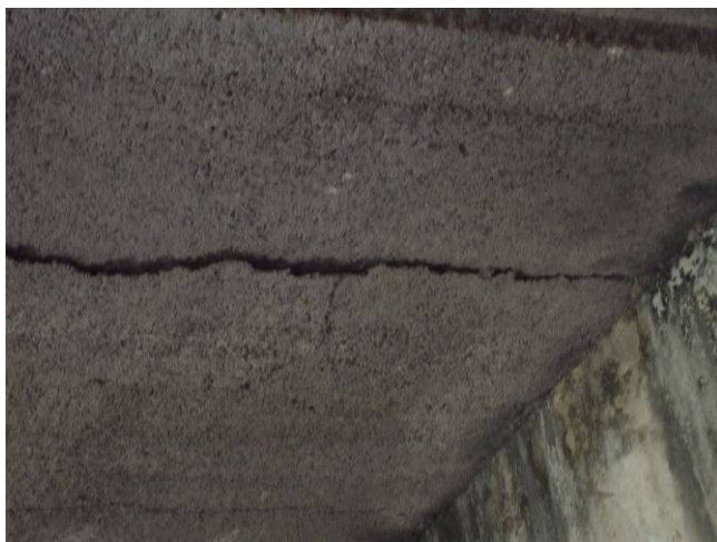
Photo C11: Typical Spancrete Slab Cracking
