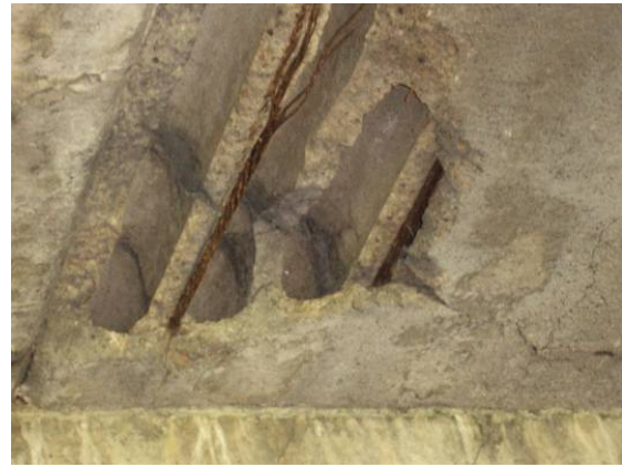
Photo # 13. Revealed voids and total failure of the prestressed wire
