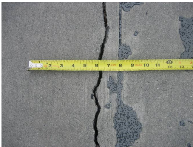
Photo C39: Slab Crack
