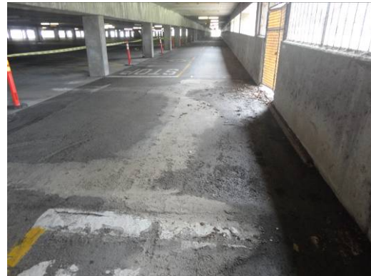
Photo # 40. Water entering parking structure from adjacent Park at Grid Line A.
