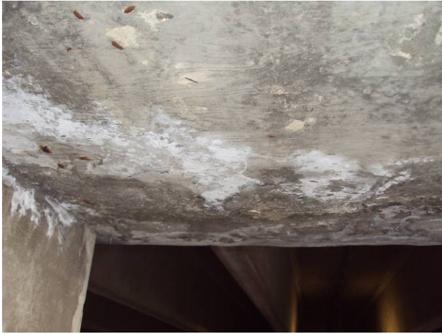
Photo B31: Lower Level Concrete Beam Distress
