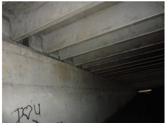
Photo C64: Double Tee Support over Channel
