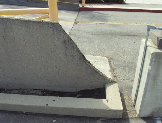
Photo B13: Precast Fascia Damage
