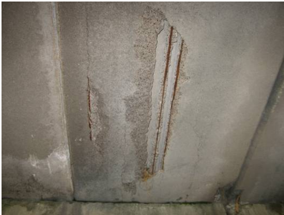
Photo # 12. Concrete spalls at the bottom of the spancrete planks adjacent to Grid Line B
