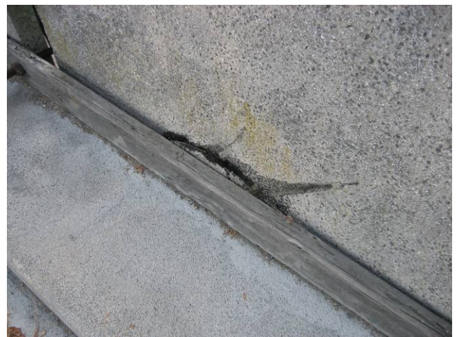
Photo C54: Damaged Wall Support
