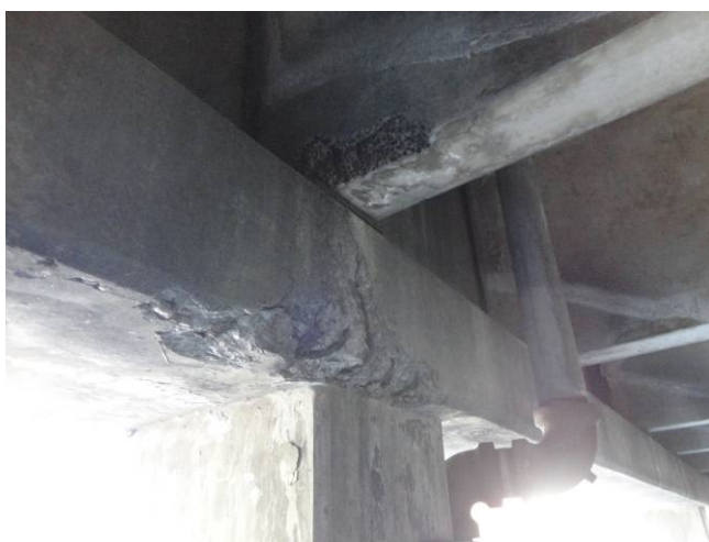
Photo C17: Girder Damage
