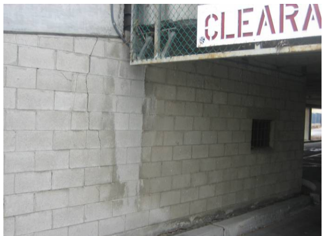
Photo C30: Crack at North Ramp Wall
