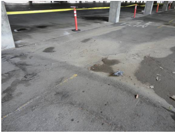
Photo # 47 Distressed asphalt overlay.
