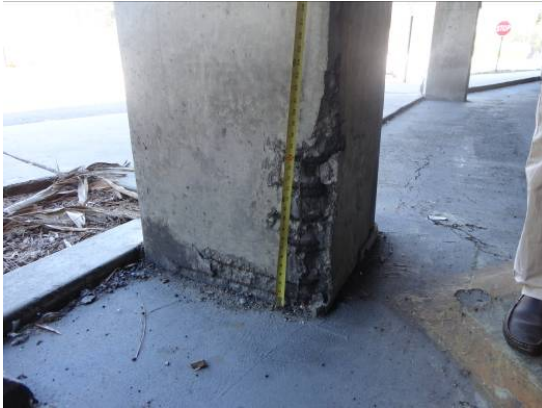
Photo # 24 Concrete cracking caused by rust of the steel reinforcing.
