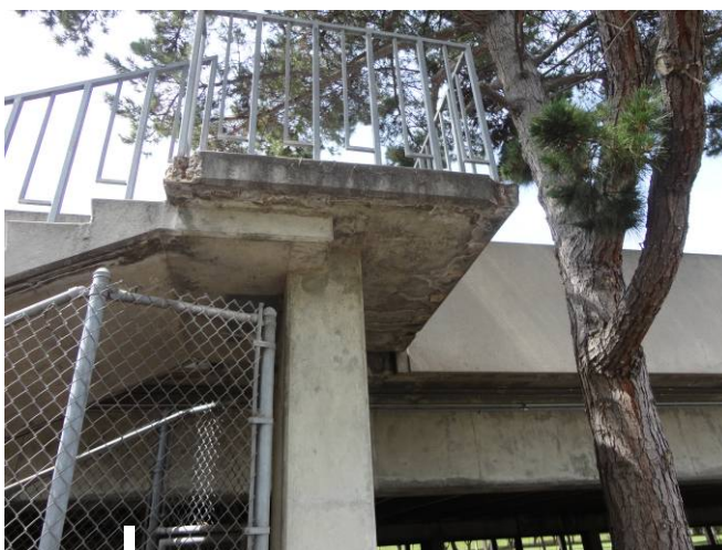
Photo A10: Stair Handrails Not Accessible
