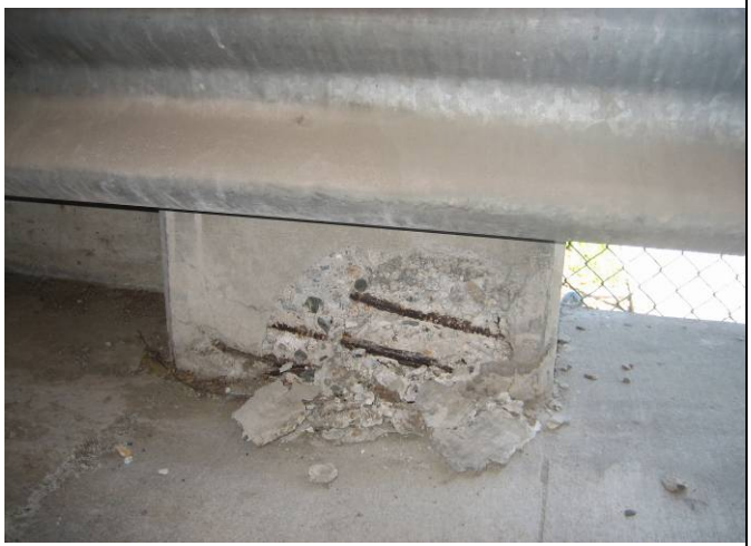
Photo C2: Column Damage
