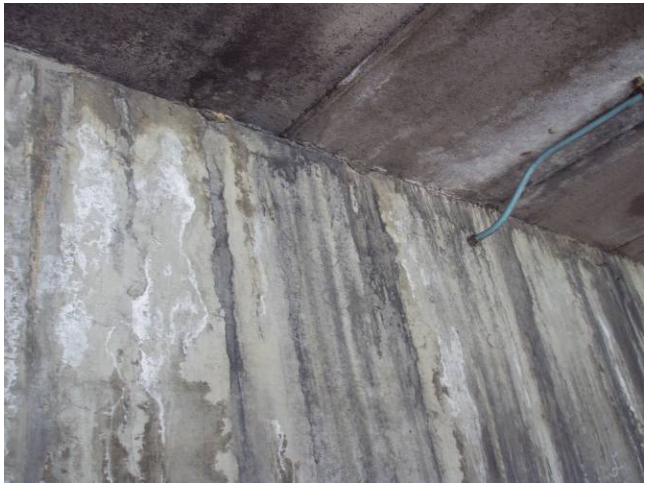
Photo B34: Lower Level Concrete Beam Distress
