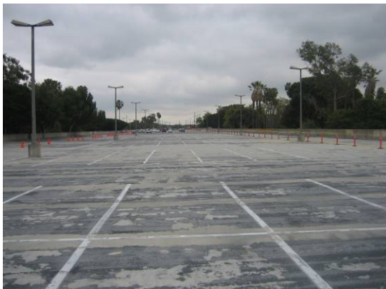
Photo # 45 Delaminating Elastomeric coating.
