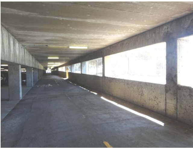
Photo C45: Short Columns at Drive Lane A-B
