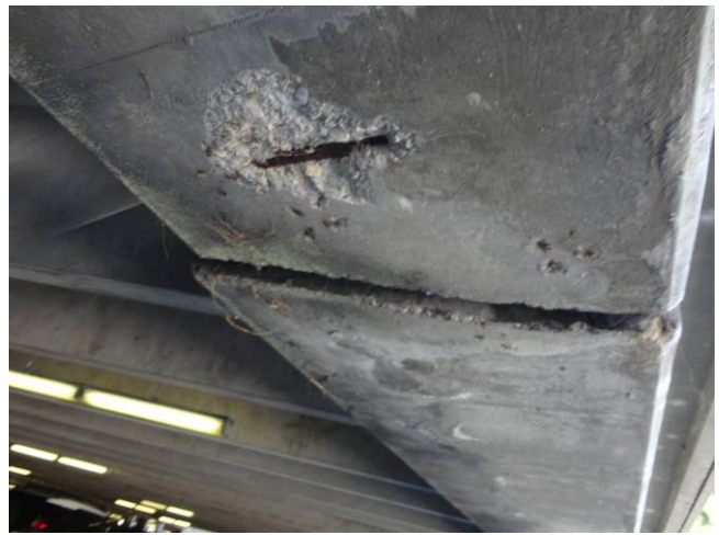
Photo C20: Girder Damage
