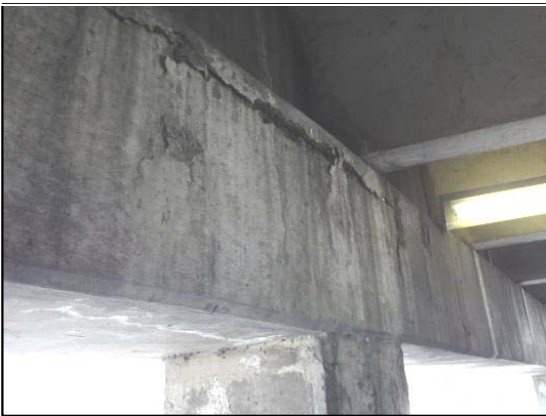
Photo # 22 Concrete cracking caused by rust of the top rebars.
