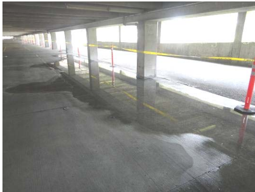
Photo # 39. Water ponding after rain at Grid Line B
