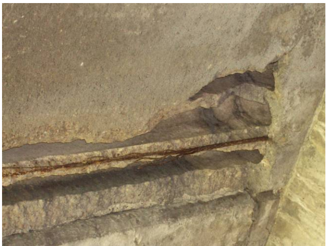
Photo B36: Hollow Core Slab Distress
