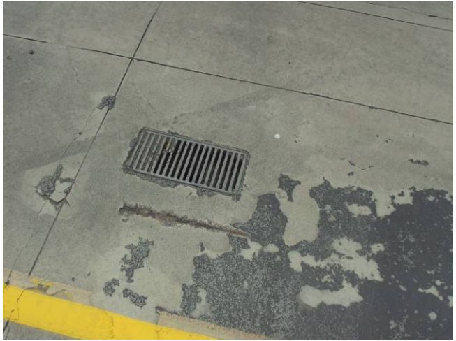
Photo B8: Clogged Deck Drain and Spalled Concrete
