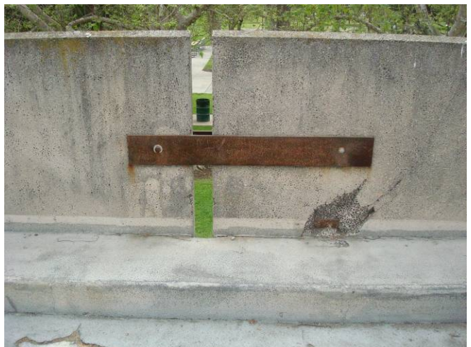
Photo C52: Damaged Wall Support
