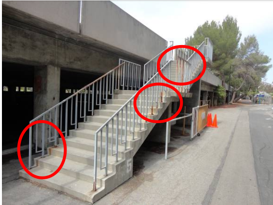
Photo # 43 Typical railing rust at stairs
