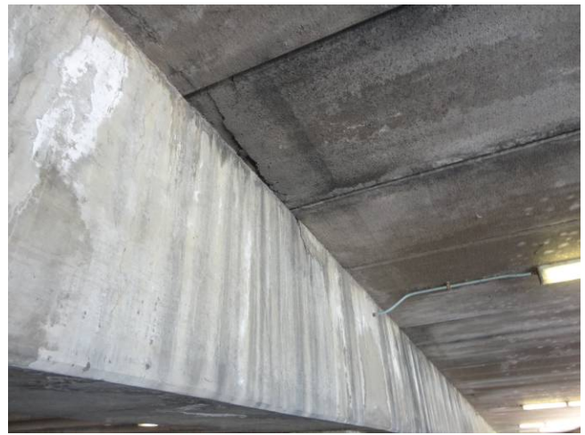
Photo C10: Typical Spancrete Slab Cracking
