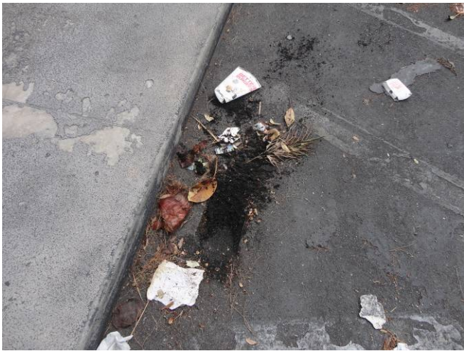
Photo B9: Clogged Deck Drain
