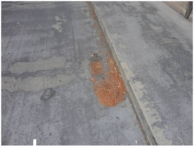
Photo B10: Clogged Deck Drain
