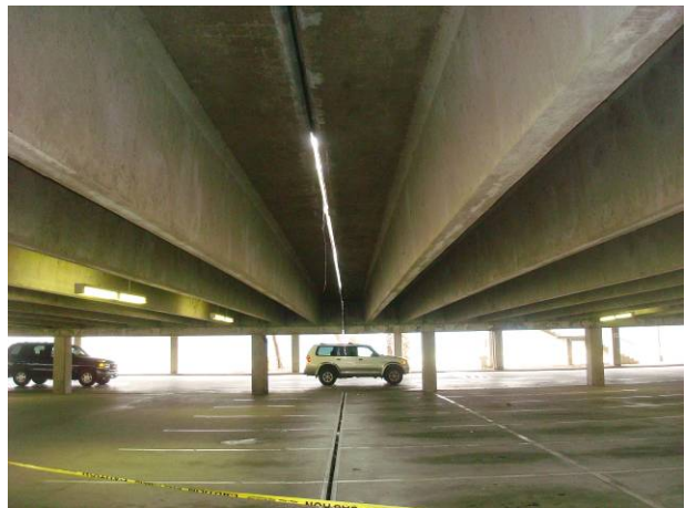
Photo # 5 Two-inch wide expansion joints separate the structure into several structural segments.
