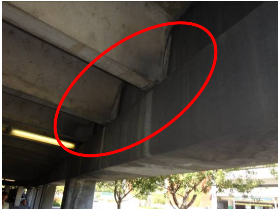
Photo # 16. Evidence of spalled concrete at the supporting ends of the 83 ft long Double Tees.
