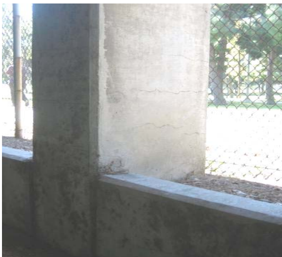
Photo C47: Cracks at Short Columns
