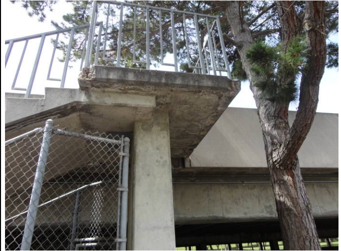
Photo B20: Stair Concrete Spalling
