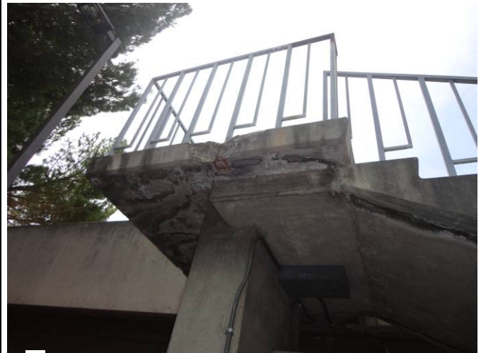
Photo B22: Stair Landing Concrete Spall
