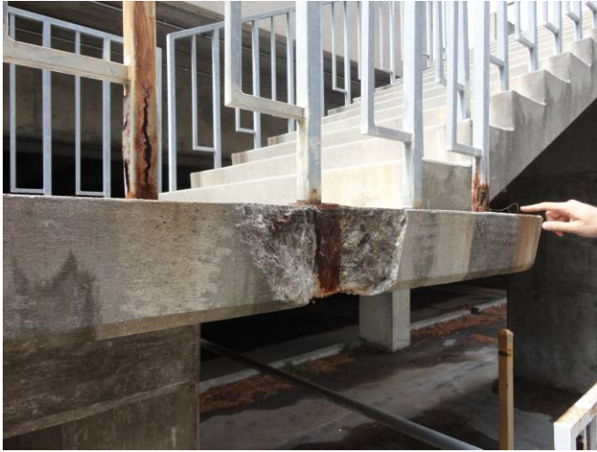
Photo B19: Stair Landing Rusting/Spalling
