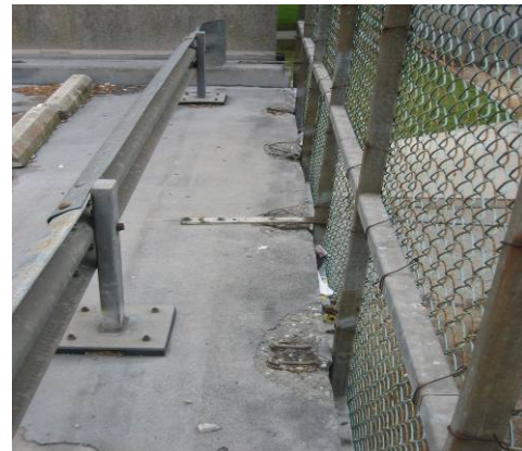
Photo # 36 Damaged screen connections
