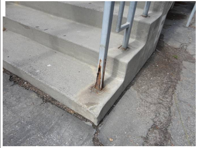
Photo B18: Stair Handrail Damage
