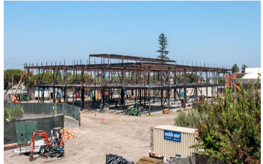
Student Services Center – under construction Anticipated completion in 2018
