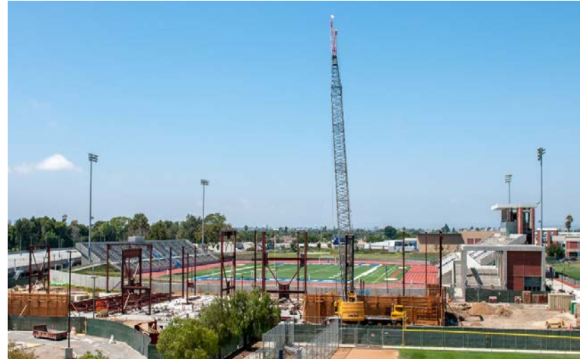
Gymnasium – under construction Anticipated completion in 2018
