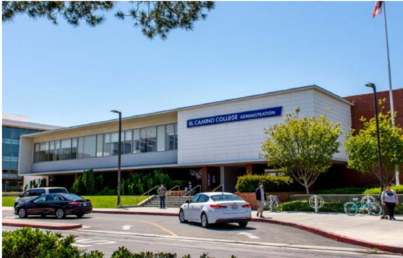
Administration Building – Will be in construction 2017–2018
